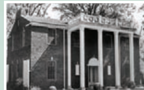
The first UA School of Nursing building in Tuscaloosa
