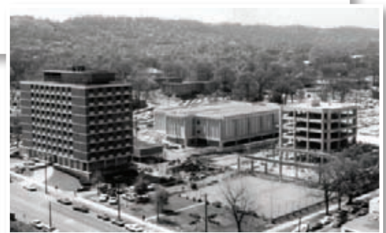
Aerial photo of the foundation of the School of Nursing building in Birmingham
